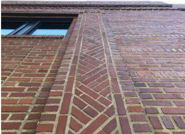
The Transformer Station has elaborate brickwork. Grant Segall/The Plain Dealer
