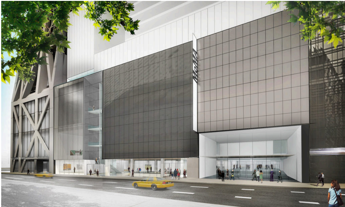
Exterior view of The Museum of Modern Art on 53rd Street.
